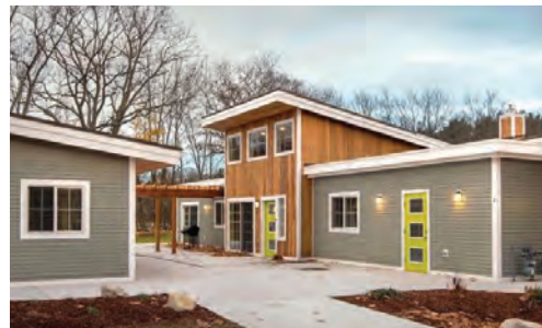
Nine-unit group home, Carlisle.
